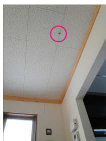
(a) Snapshot of sensor on the ceiling.
